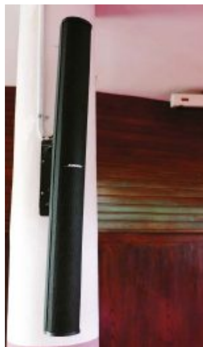
L-R MA12EX Panaray column speakers are fixed to rising columns by Bi-Pivot brackets
